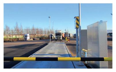
1. Wait in front of the boom until the previous vechile has left the weighbridge and the boom is in the upper position. Follow the display messages if the boom does not open, and act according to the instructions given on the display.
